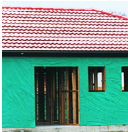
"Wrapped and sealed in a barrier"
