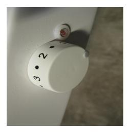
**TEI 1** (Manual Thermostat) – this thermostat is located on the side of the radiator and can be manually adjusted to regulate the temperature within the room.
