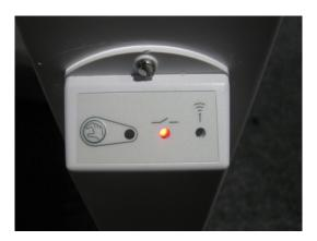
When it stops a red LED light will light up on the receiver, indicating that now the radiator is ready to heat up.
